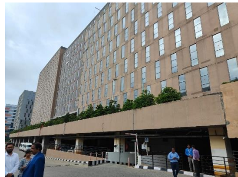
External View of Subject Property
