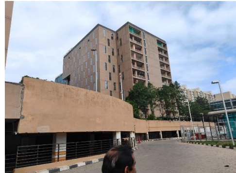
External View of Subject Property
