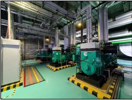
View of DG Room
