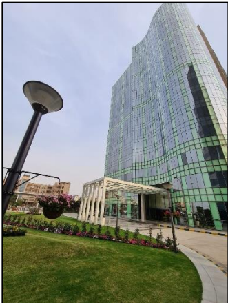
External View of Block 5
