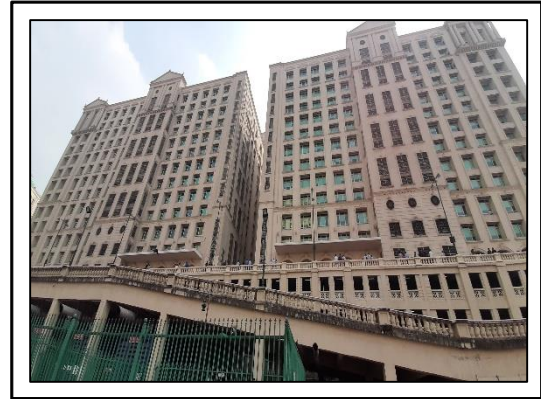
Building (A & B) – Rear View
