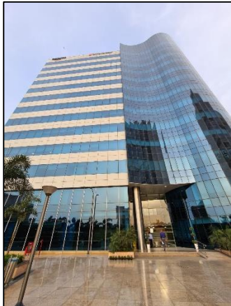
External View of Block 3
