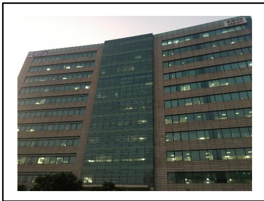
Front view of Tower 1
