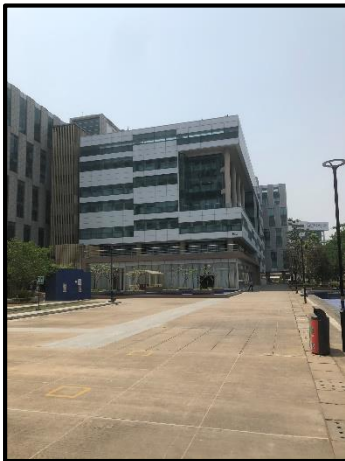
View of Tower B2
