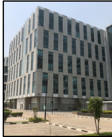
View of Tower B1
