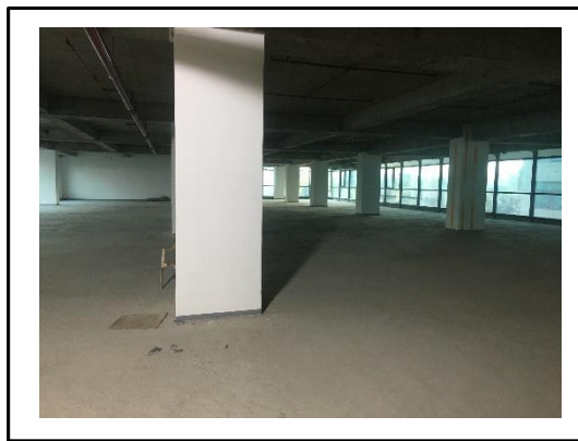
Internal view of under construction Tower 11
