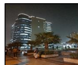
External View of Subject Property (Block - 3)
