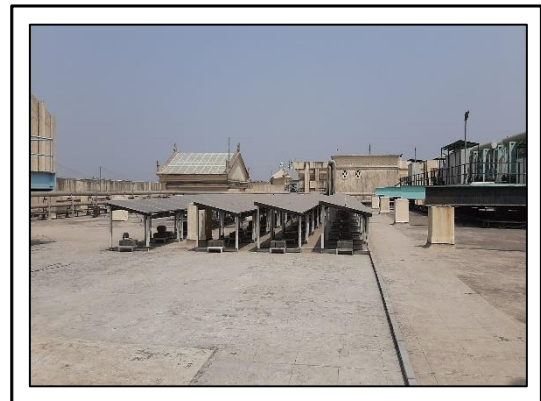
Building Terrace Area
