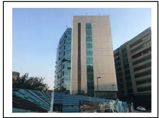
External view of under construction Tower 11
