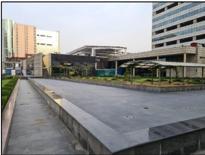
External view of Block 7
