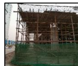
Under Construction Block 8 (Amenity Block)
