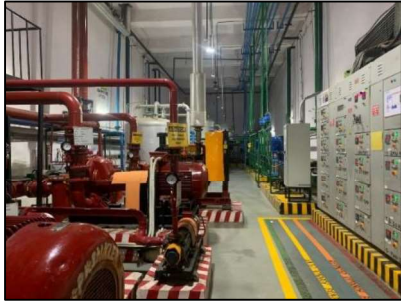
Internal View of Pump Room
