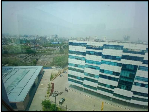
View of Tower G1
