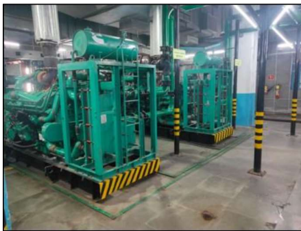
Block 9 & 10 DG Room
