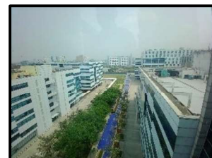
Open space inside the Subject Property
