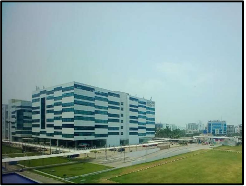
View of Tower G3
