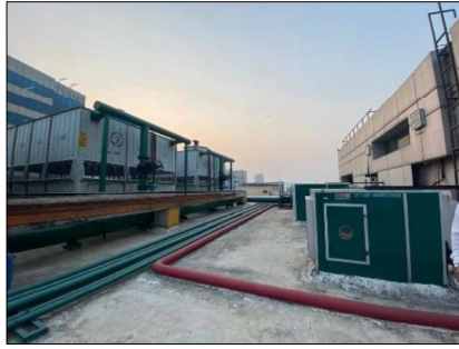
View of Tower 4 Terrace
