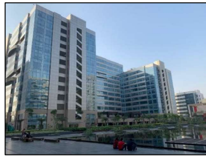
External View of Tower 4, 5, 6
