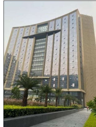
External View of Tower 11
