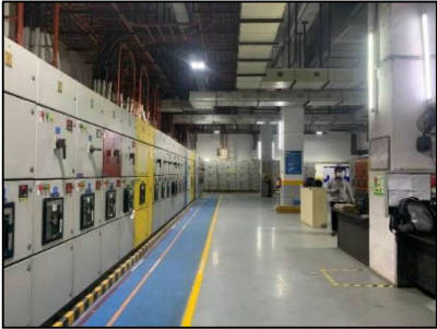
Internal View of LT Panel Room
