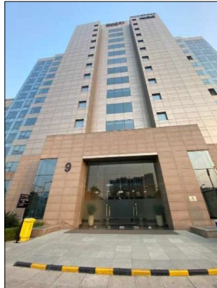
External View of Tower 9
