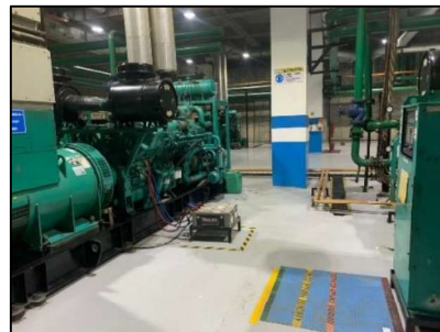
View of DG Room
