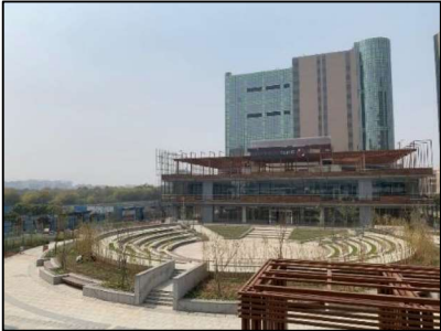
External view of Block 7
