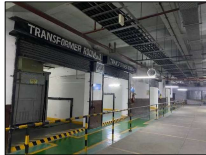
View of Transformer Room Tower 8, 9, 10
