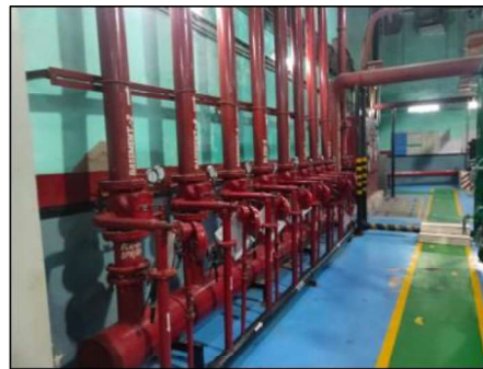
WTP & Fire Pump Room
