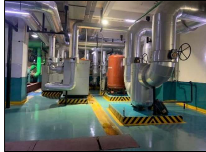
Internal View of Plant Room Tower 4,5,6
