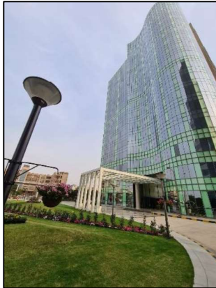
External View of Block 5
