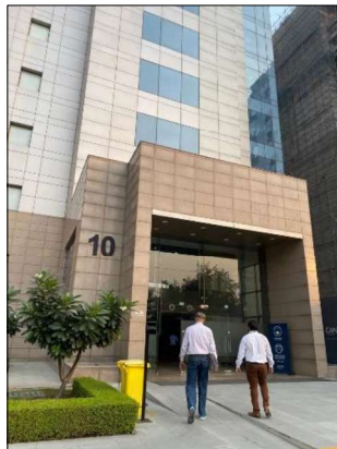
External View of Tower 10
