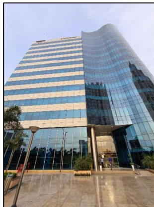
External View of Block 3
