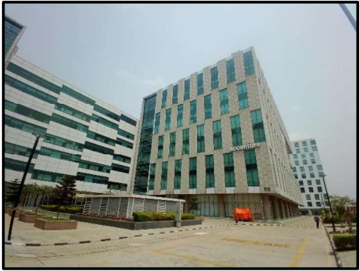
View of Tower B2
