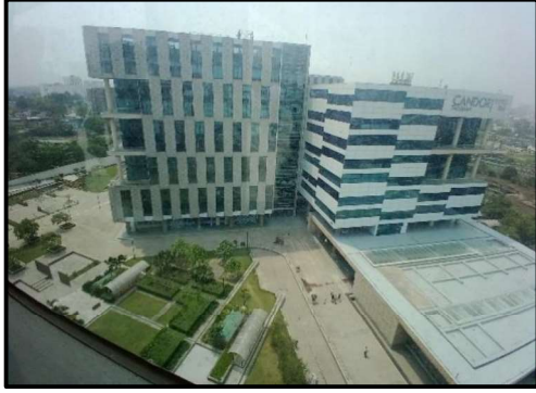
A Block of the Subject Property
