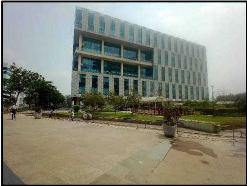
View of Tower B1
