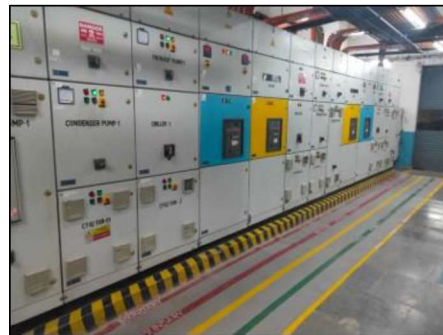
Block 7, HVAC Room
