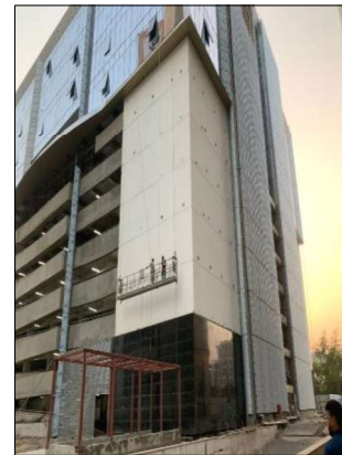
View of Tower 11A (UC)
