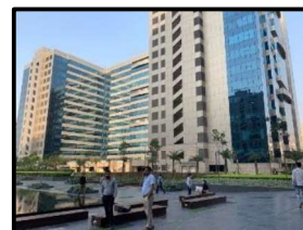
View of Tower 4, 5, 6
