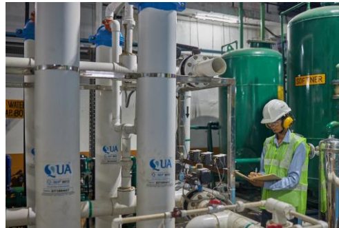
STP Plant with Ultra-filtration
