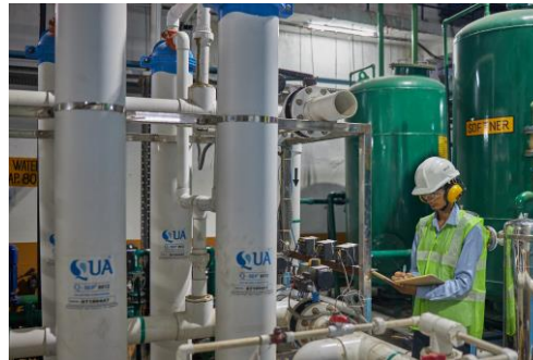
STP Plant with Ultra-filtration
