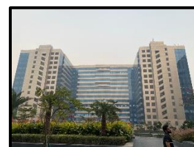
View of Tower 4, 5, 6
