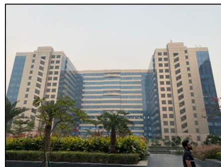
External View of Tower 4, 5, 6
