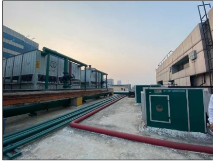
View of Tower 4 Terrace
